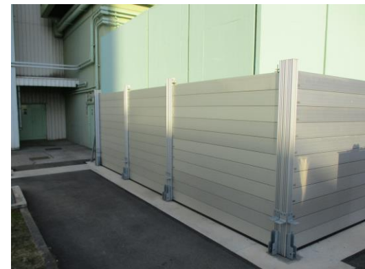
Flood retaining walls
